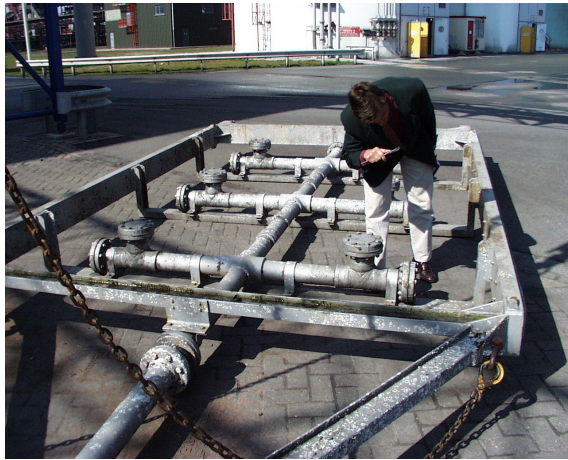
Figure 13 Dosing rack at Maasvlakte power station
