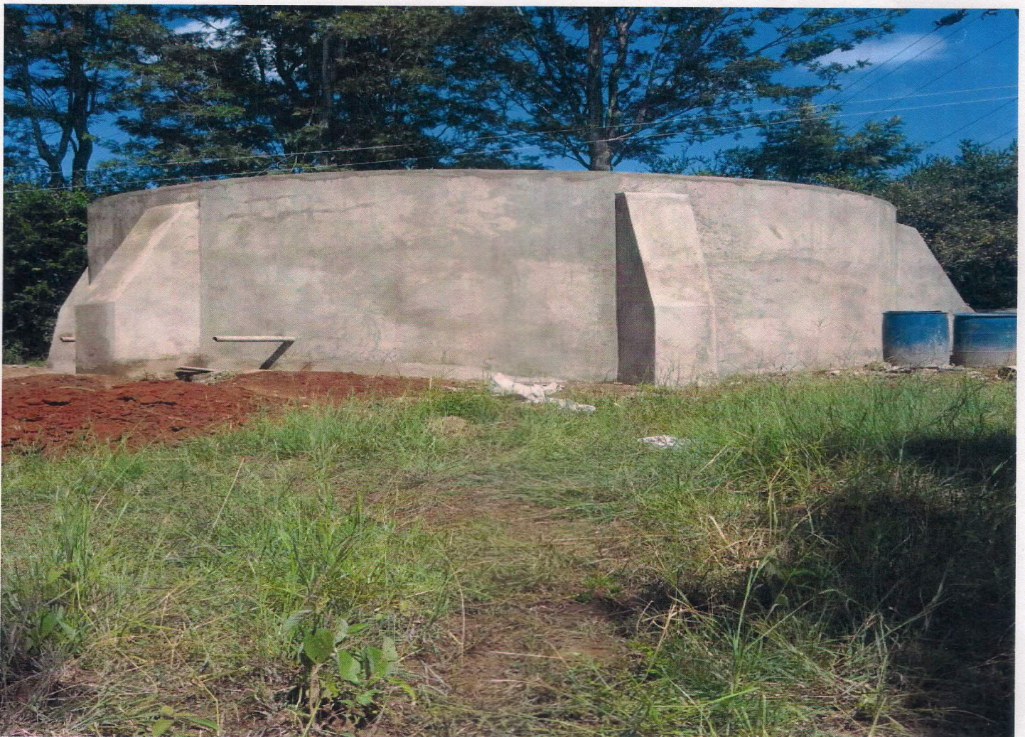
DISTRIBUTION TANK AFTER REHABILITATION
