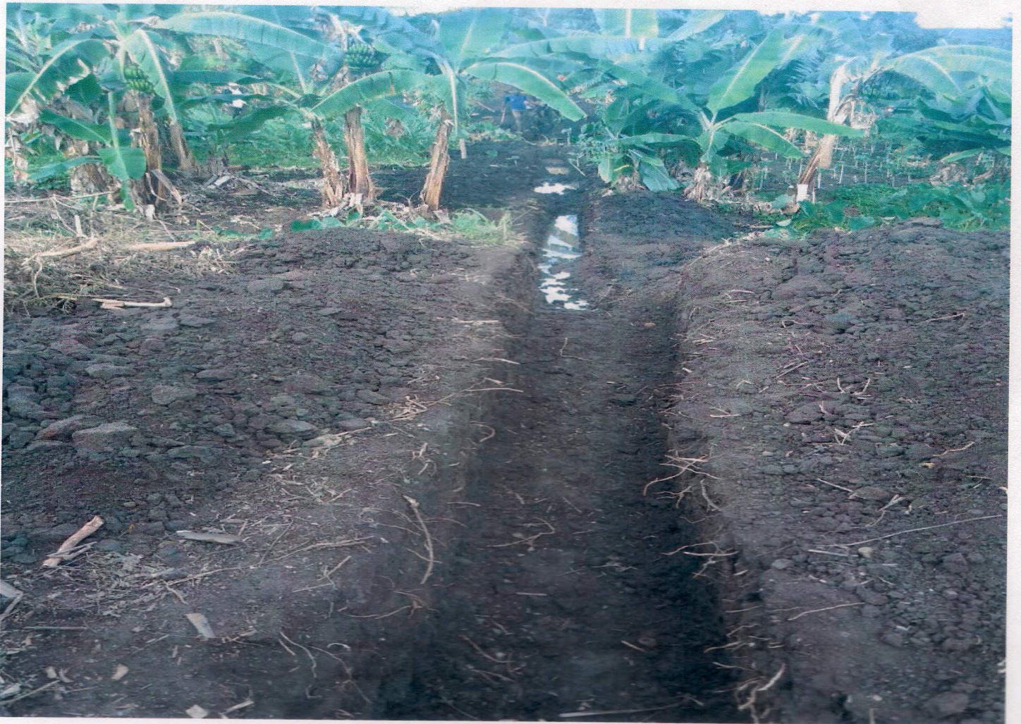
TRENCHES FOR LAYING HDPE PIPES
