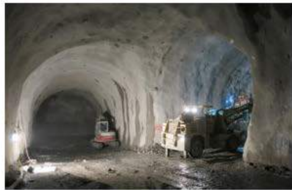
Access tunnel OVW II – under construction
